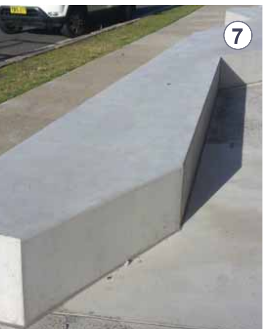
Off form concrete seats
