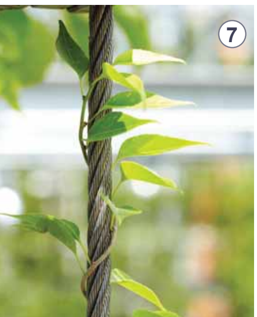
Steel Cables for Vine Growth
